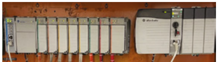
Allen Bradley ControlLogix PLC using Allen Bradley CompactLogix remote rack, at McAlpine's Rangiora.
